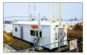
Units for gas treatment, reduction and distribution are aimed for treatment of fuel gas for gas piston and gas turbine drives of compressor stations, power stations and other consumers.
