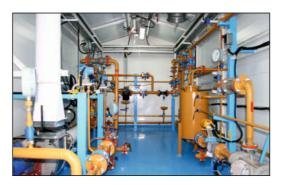
Units for oil quality parameters metering are aimed for automatic determination of physical and chemical parameters of oil quality as per GOST R 51858-2002, automatic and manual oil sampling for further oil quality analysis.
