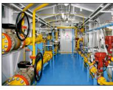
Gas metering systems are aimed for determination of quantity, quality parameters, automated metering of natural and associated gas.
